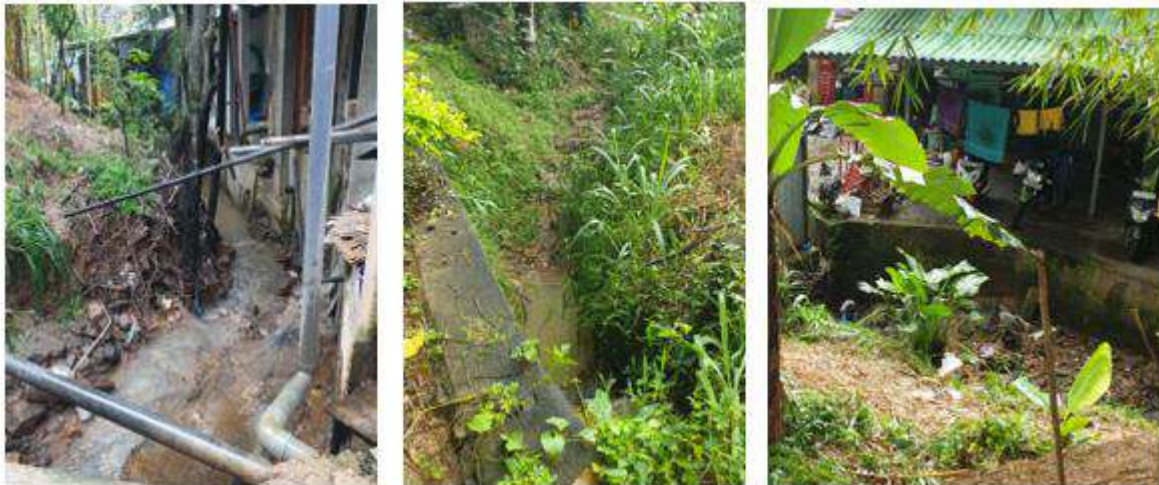
Figure 02: Hotels and households have connected their sewer lines into nearby streams and canals
