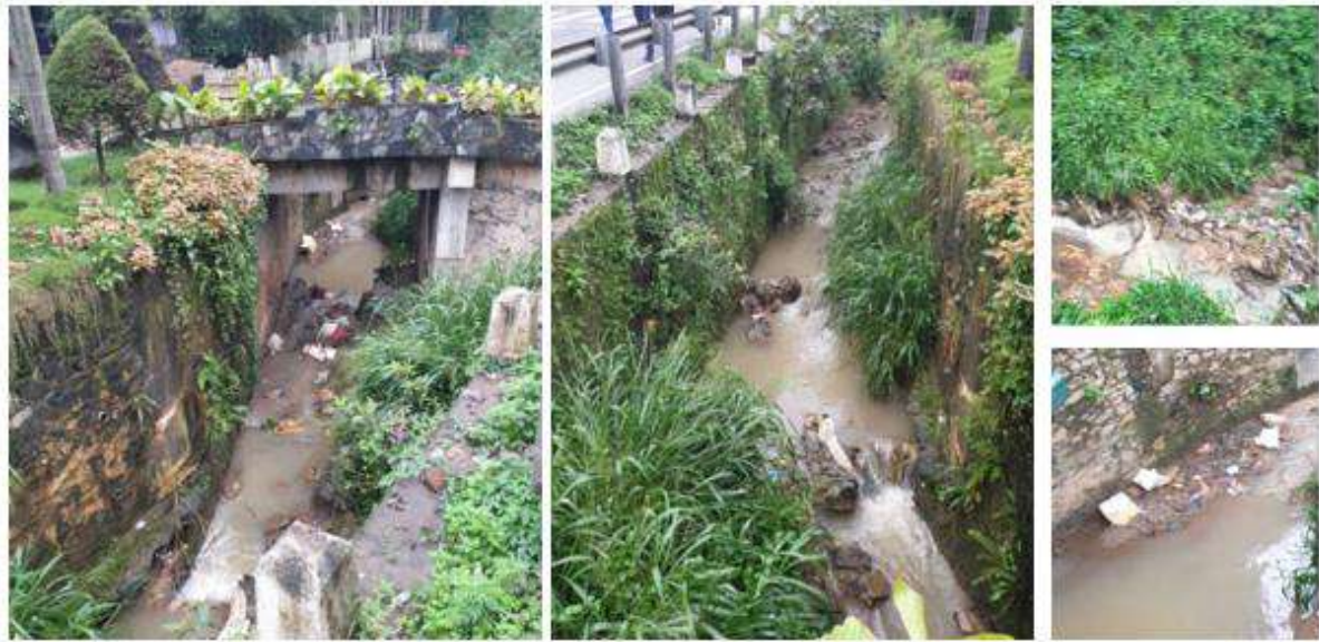
Figure 03: The main canal is extremely polluted with raw sewage, and the flow is interrupted by solid waste dumped into the canal
