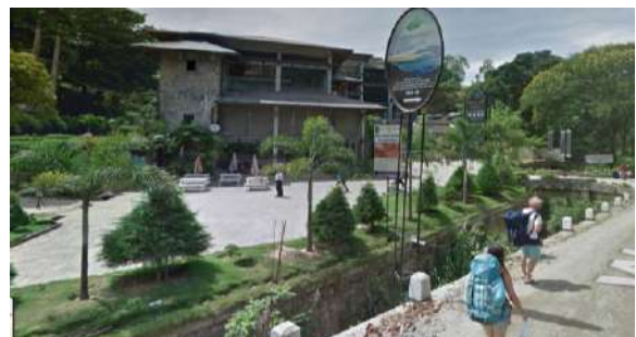
Figure 2-3: Existing storm water drain running via the Ella city center
