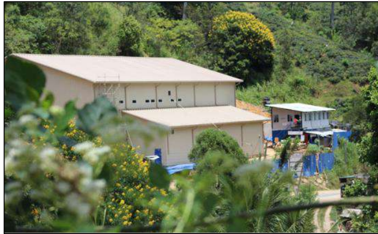
Figure 02: Badulla-Hali Ela-Ella Integrated Water Supply Project
