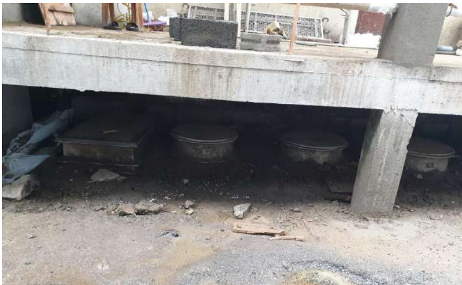
Figure 04: Some hotels have septic tanks, but without any soakage pits. These tanks are either emptied by gully bowzers or simply overflow/emptied into the nearby streams or canals
