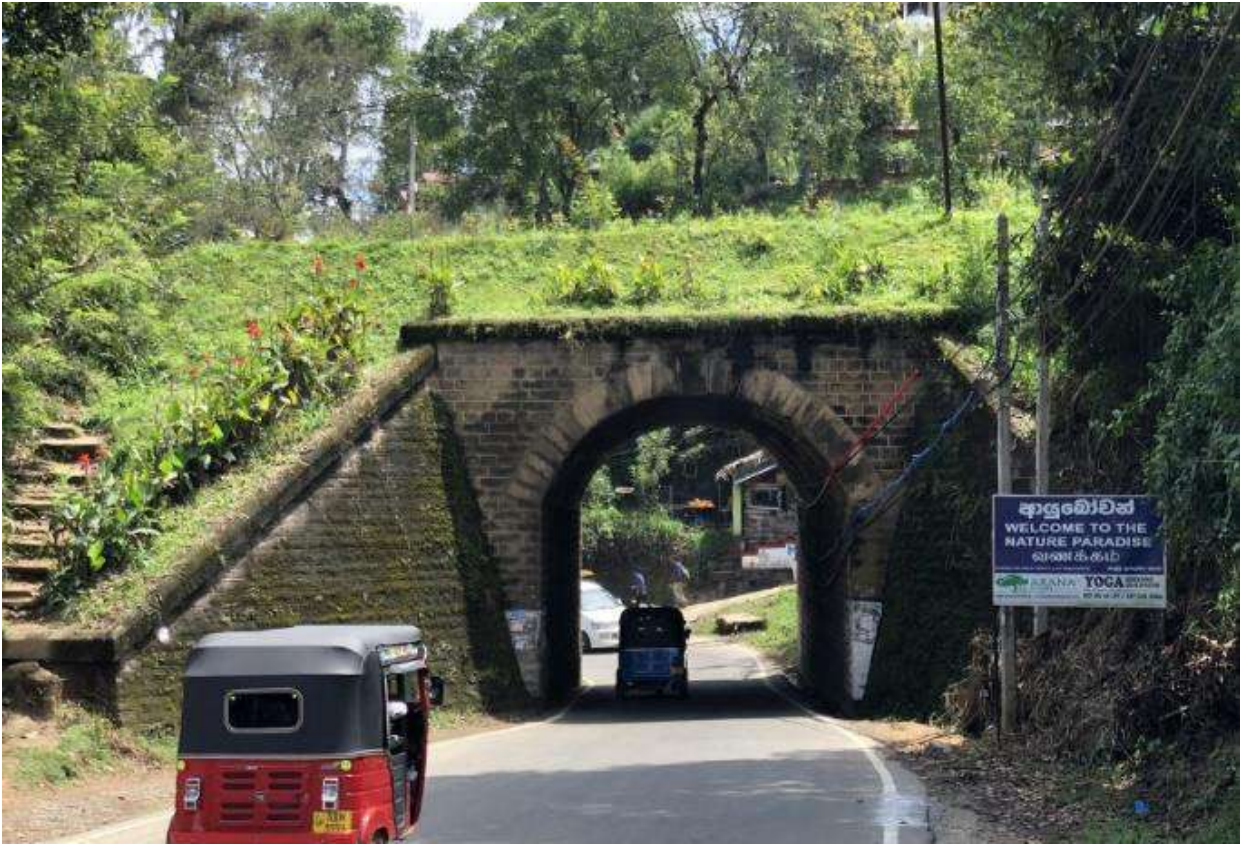
Figure 3-1: Existing tunnel at Ella
