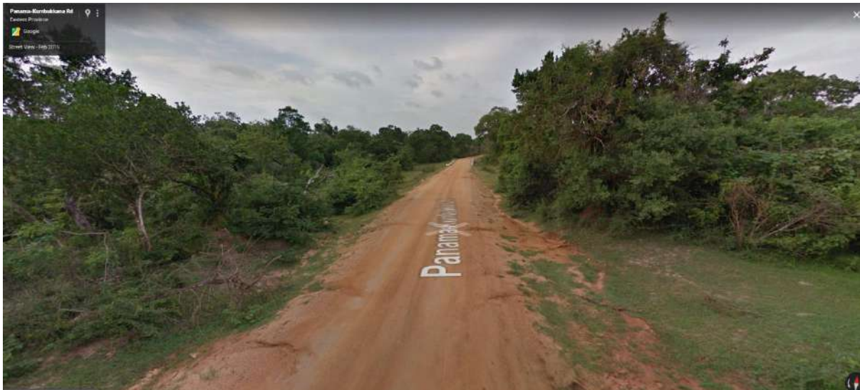
Figure 8 5: Road surface of B 355 road
