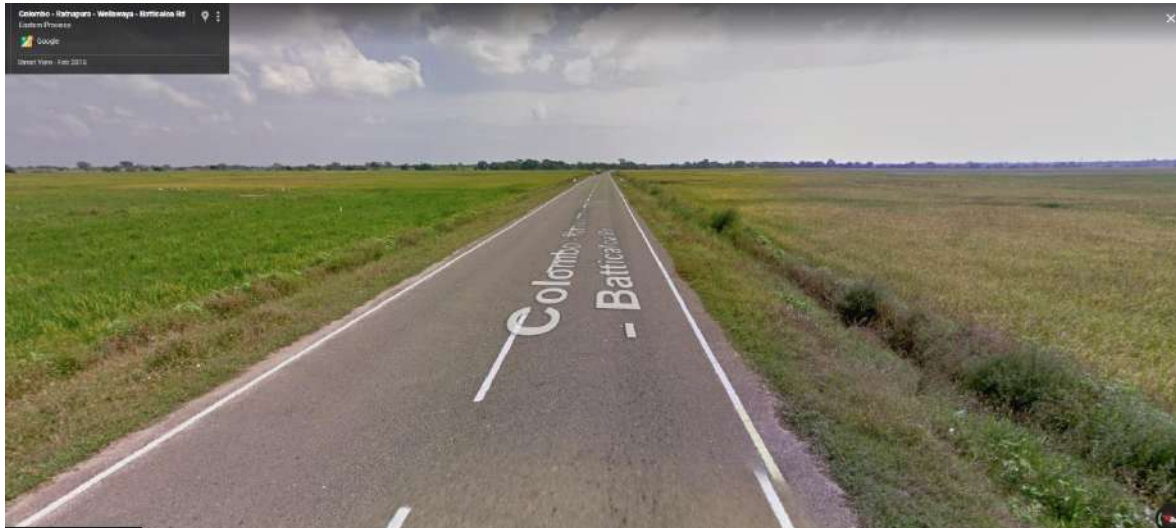
Figure: Road surface of A 04 road
