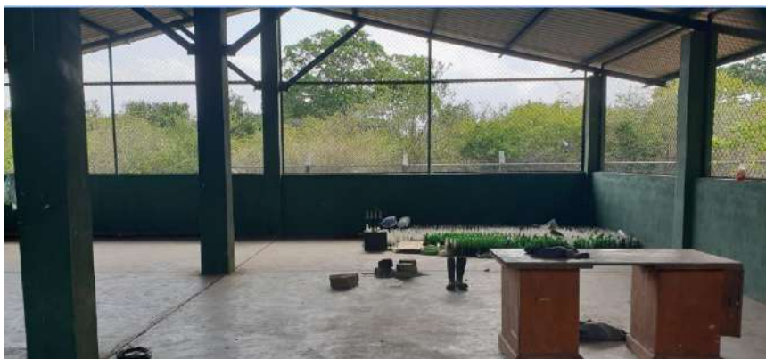
Figure: Sorting and Storage area is not properly utilised
