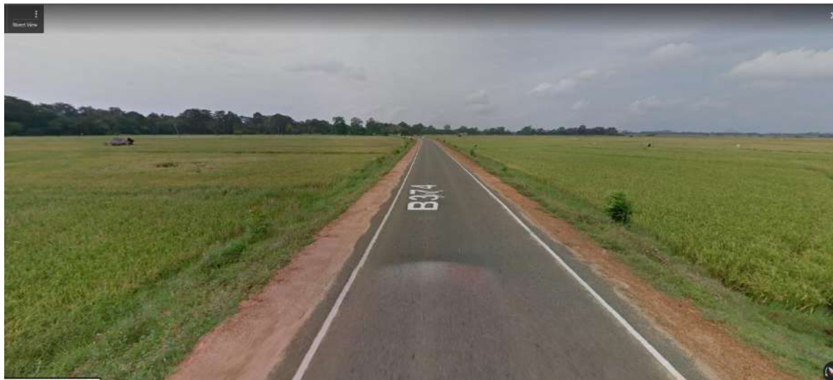
Figure: Road surface of B 374 Road
